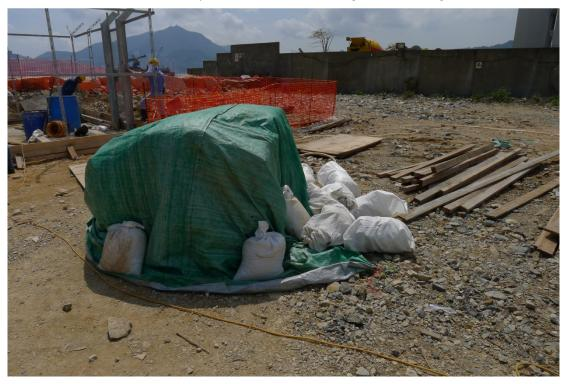
*Photo 3 – Dusty construction material has been well covered by tarpaulin sheet.*
