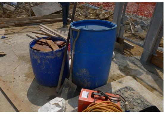
*Photo 4 – Contractor has been advised to cover the water bucket after use to prevent mosquitos breeding.*
